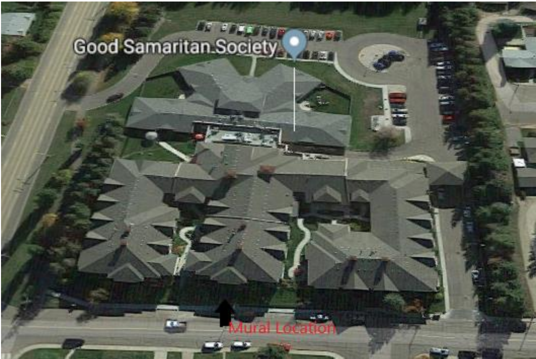
Image 1: Aerial View of GSS Building and Mural Location (55 th Avenue at bottom of image)
