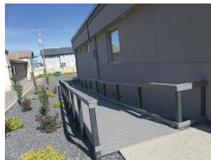
48th Street, Ramp
