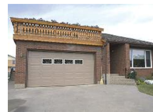
Old Town, Roof Top Terrace
