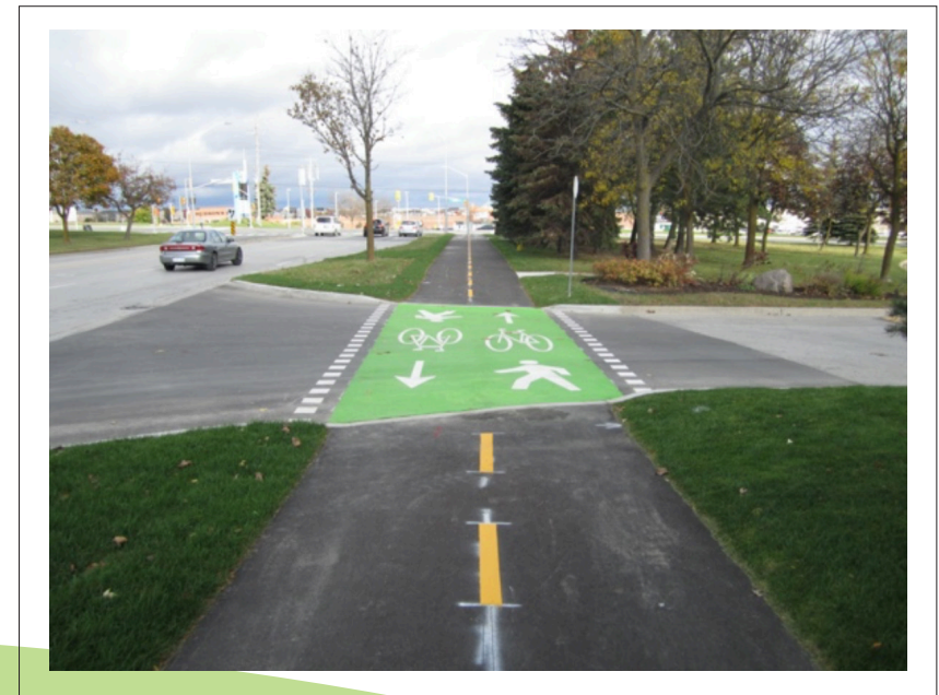
FIGURE 4.9: COMBINED CROSSING WITH GREEN PAVEMENT MARKINGS
