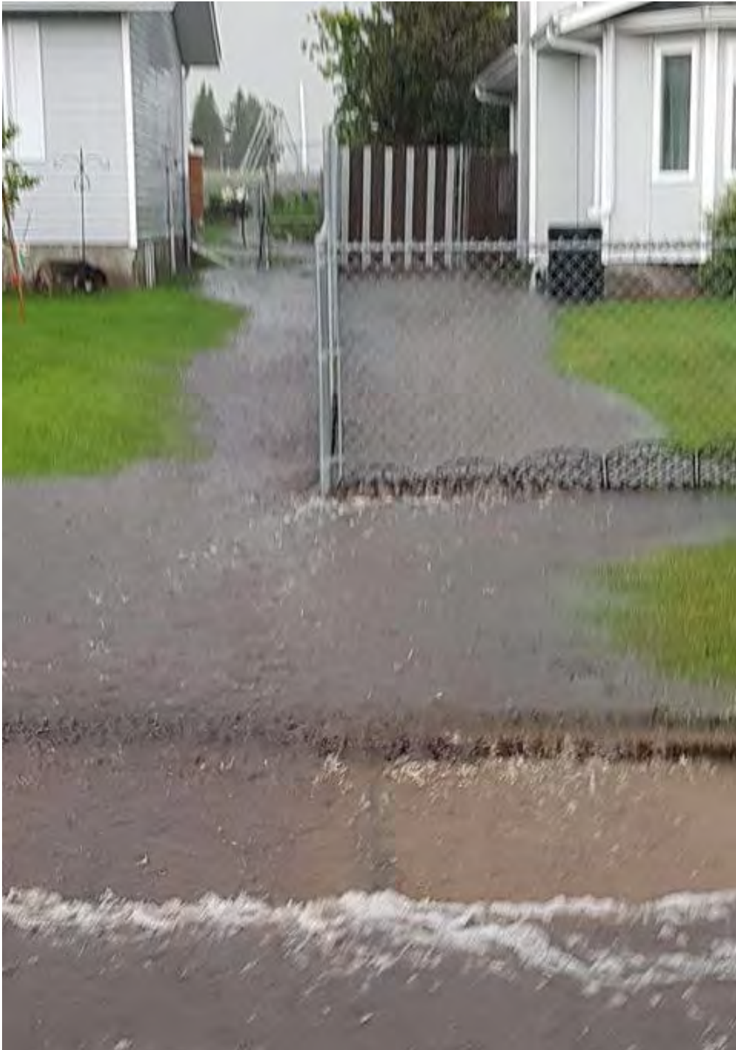
Figure D- 14: Area H – 57 Avenue just west of Glenwood Crescent, looking north between two properties that overlook the school playground to the back, showing significant amount of surface drainage flowing from the school yard towards 57 Avenue. July 15, 2019
