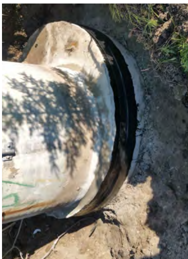
PHOTO OF MANHOLE JOINT WRAP WITH 9\"/>
