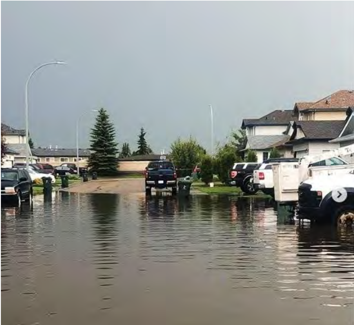
Figure D- 4: Area B – Egerland Place bend, looking east towards Egerland Place, showing significant ponding on the road. July 15, 2019
