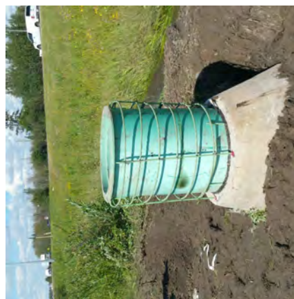
PHOTO OF MANHOLE CHIMNEY REBAR
