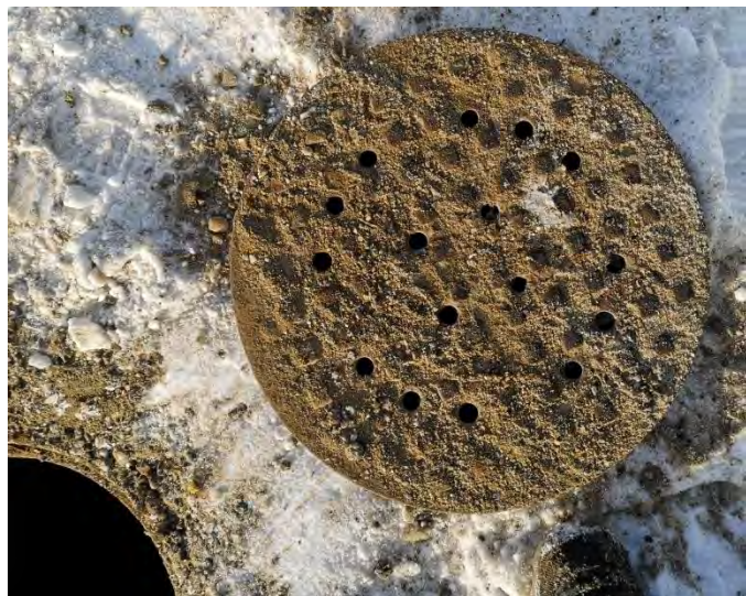
Figure 6-29: Catchbasin-Type Cover on Sanitary Manhole at 44/46 Boulder Boulevard
